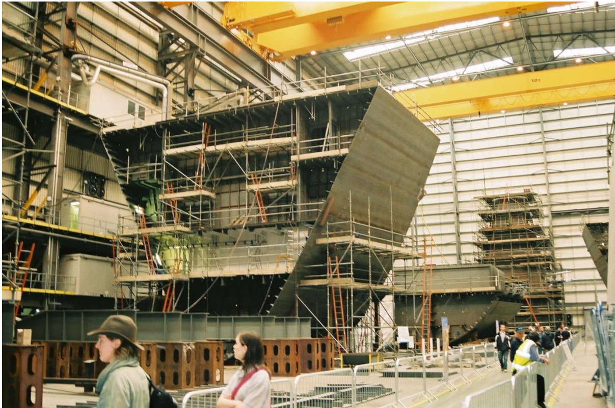
Figure 13. Modular blocks of HMS Dauntless under fabrication at HMNB Portsmouth. Image courtesy Adrian Jones.
