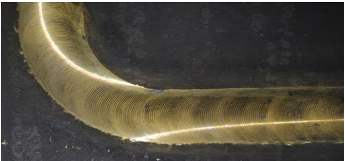
Figure 7. View of a 4mm thick plate lap welded onto a simulated damaged hull plate, under water
