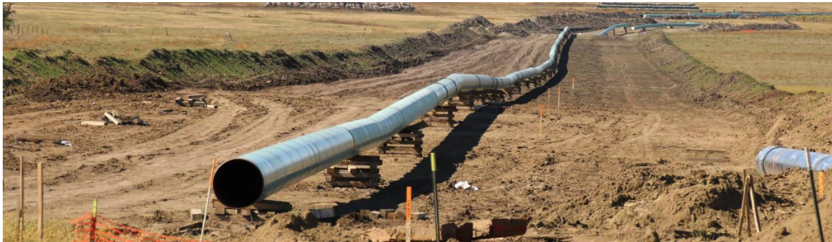
Figure 21. Conventional pipeline installation.
