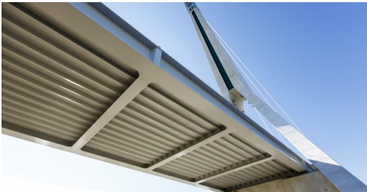
Figure 14. Steel bridge decking
