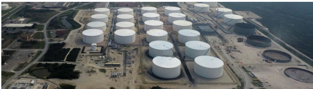
Figure 15. Large storage tanks
